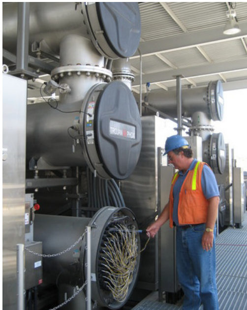
Figure 3 GWRS ultraviolet reactor system (Photo Credit: Gina DePinto)
