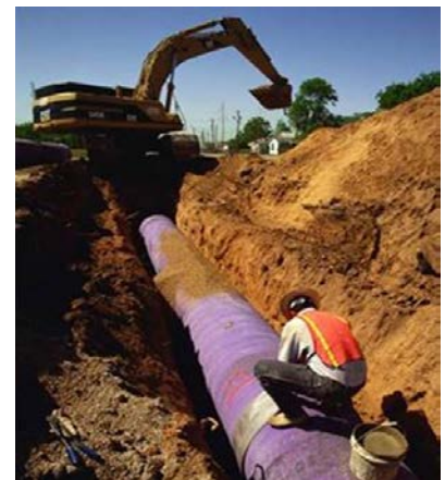
Figure 2-2 36-inch CSC 301 purple mortar pipe, San Antonio Water System (SAWS). (Photo credit: Don Vandertulip)
