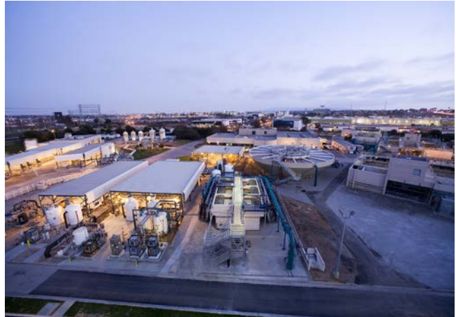
Figure 1 The Edward C. Little Water Recycling Facility is located in El Segundo, California
