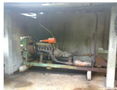
Figure 1 Composition of the system at Sam Pran (from top to bottom): channel digester and solids drying beds for use as fertilizer, aeration tank, water hyacinth pond, and biogas-fueled generator.
