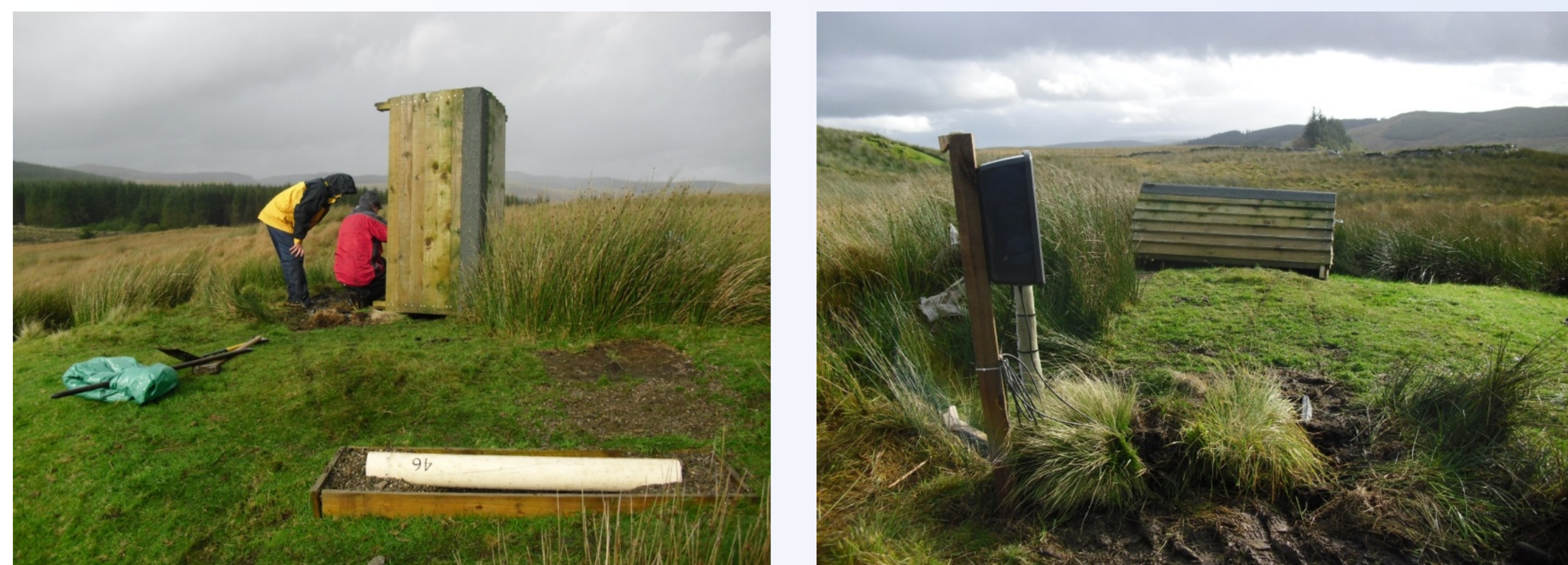
Figure 1: Installation of Channel 1 (North) induction coil at Eskdalemuir [55.314° N, 356.794° E] in the Scottish Borders, UK. Left image: The coils (white tube, foreground) are located in a rural valley (background), protected from wind, rain and snow under a non-magnetic wooden cover (shown upright in midground). Right image: Looking eastward to the enclosed coil under wooden cover. The signal is digitized close to the coil before being converted to a higher voltage at a breakout box (mounted on the post) and sent to a logging computer in a vault approximately 150m away.
