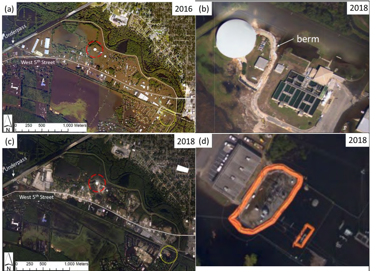
Figure 2-9. Lumberton water plant and an electrical power network substation in the leveed area of Lumberton that flooded in: (a) 2016 from Hurricane Matthew (NOAA, 2016) with (b) Close-up of Lumberton Water Plant, and (c) 2018 from Hurricane Florence (NOAA, 2018) with (d) Close-up of the electrical substation.
