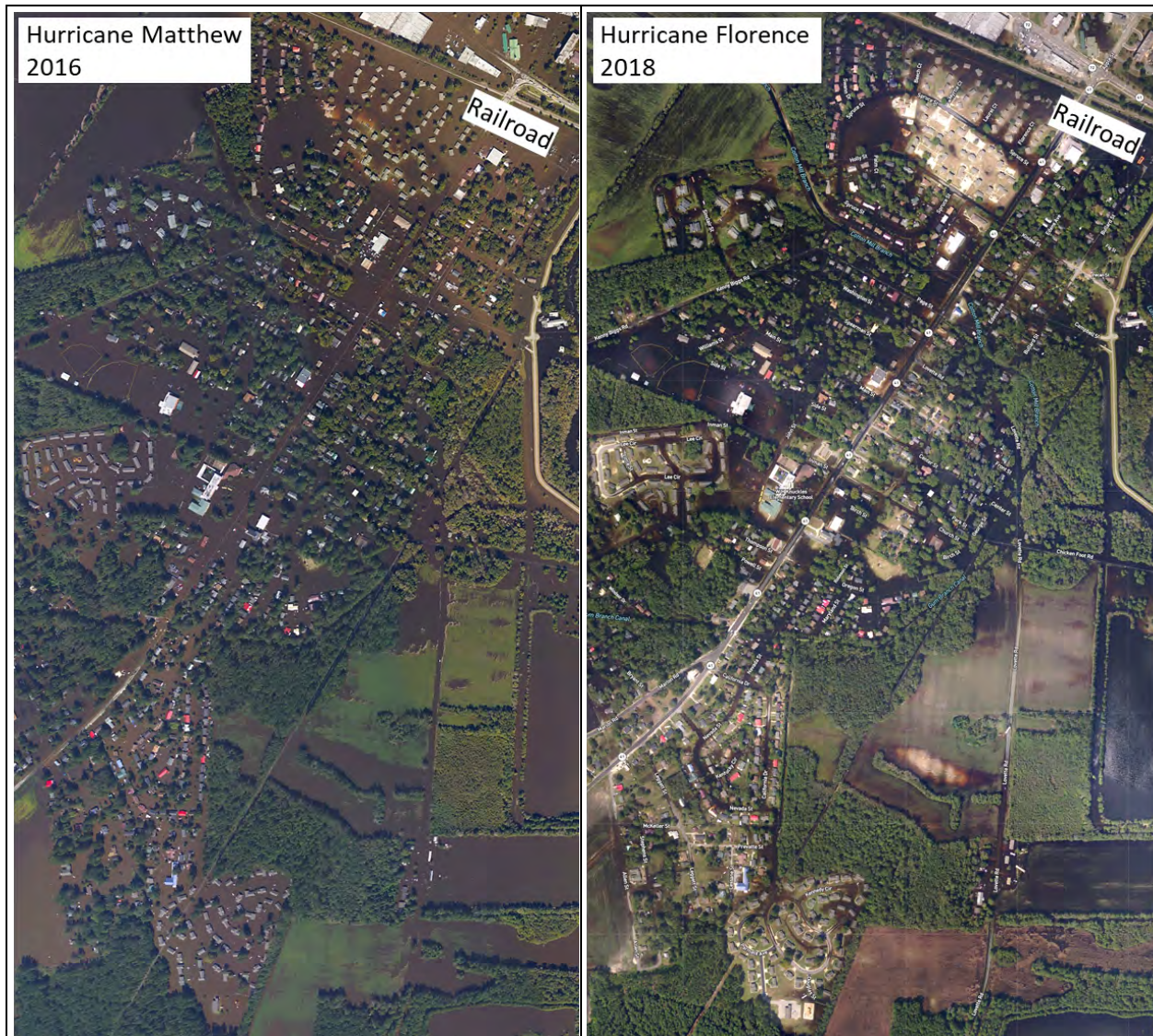
Figure 2-1c. Residential area South of the Lumber River and railroad indicated by (c) in Figure 2-1. Imagery collected following Hurricane Matthew (NOAA 2016) and Hurricane Florence (NOAA 2018) has been edited to show flooded areas more clearly.
