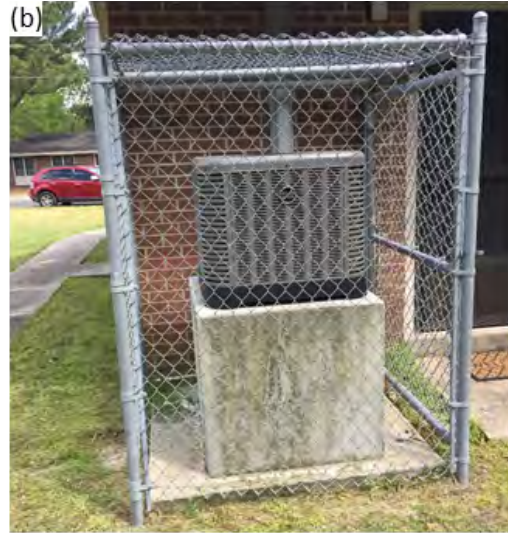
Figure 2-10. Examples of visible individual-level mitigation efforts in Lumberton implemented before the 2018 Flood; (a) Temporary perimeter flood protection around international retailer building (NOAA 2018); (b) Elevated air conditioning condensers in a public housing complex.
