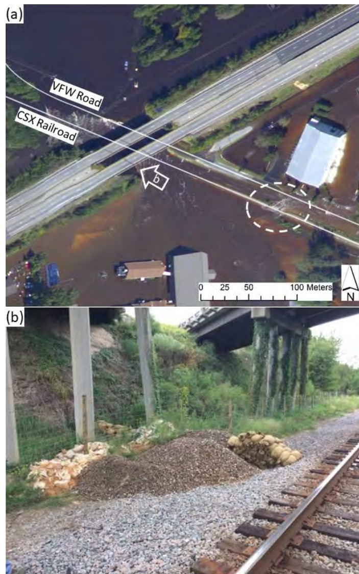
Figure 2-6. I-95/CSX Underpass seen in 2016: (a) from above; (b) from underneath, with flood prevention set in place. (NOAA, 2016). Photograph shown in (b) reproduced with permissions from van de Lindt et al., 2018.
