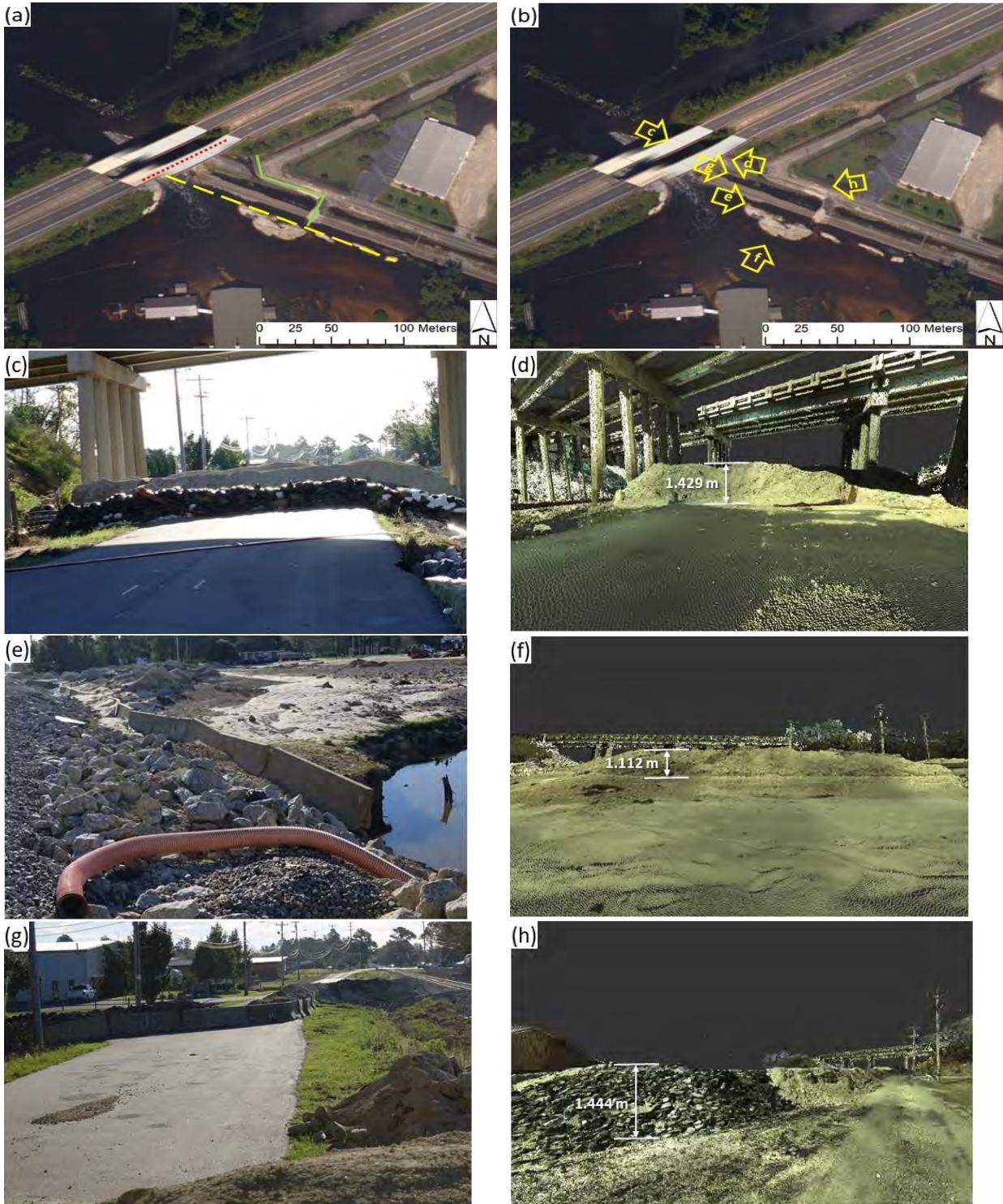
Figure 2-7. Berm system deployed before Hurricane Florence: (a) Aerial overview with three berm sections marked (NOAA 2018); (b) Aerial overview with image locations and orientations (NOAA 2018); (c) Primary berm section; (d) LiDAR scan of primary berm section; (e) Secondary berm section; (f) LiDAR scan of secondary berm section; (g) Tertiary berm section; (h) LiDAR scan of tertiary berm section.
