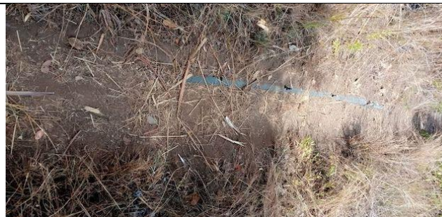
Existing inferior pipes – Class A PCV pipes
