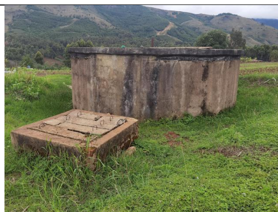
1980s Existing storage tank
