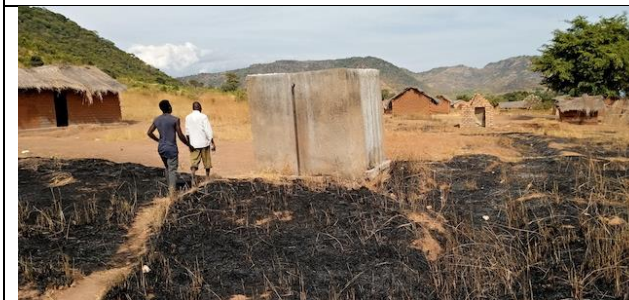
Only small storage tank at Kizumbi village
