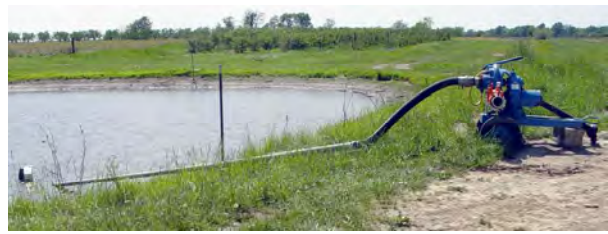
Figure 3-6-A. Portable pump at irrigation pond.
