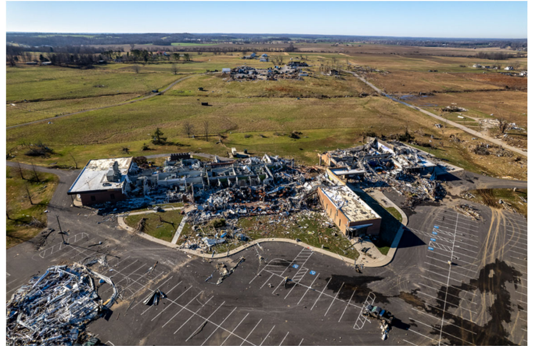
Aerial view of the UK Research and Education Center after it took a direct hit from a weekend tornado. Photo by Matt Barton, UK agricultural communications.
