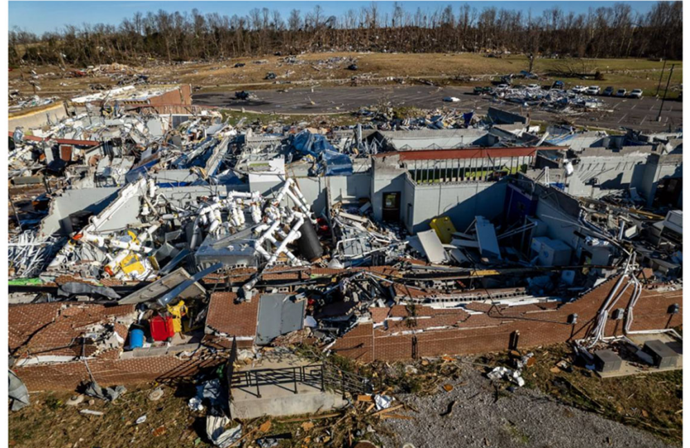
The Grain and Forage Center of Excellence at the University of Kentucky Research and Education Center in Princeton was damaged by a powerful tornado last weekend.. Matt Barton | UK College of Agriculture
