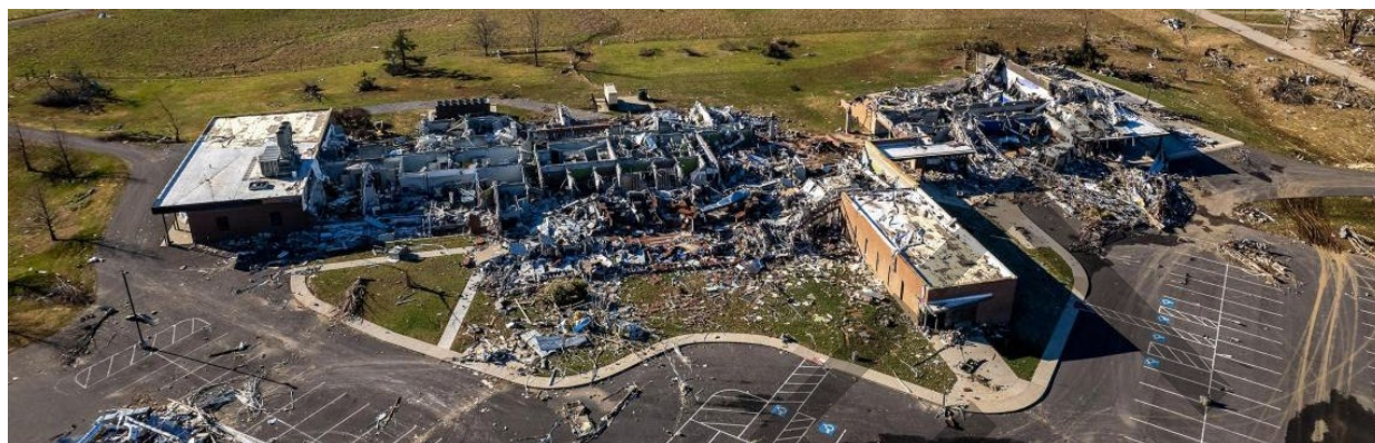
Figure 3-83: UK Grain and Forage Center of Excellence Following the Tornado
