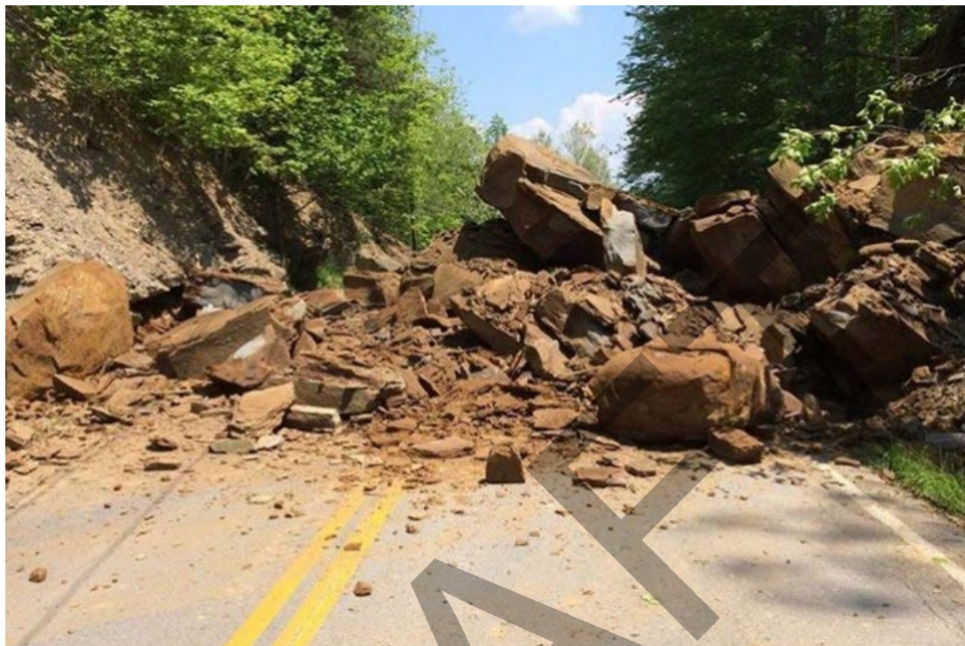
Figure 3-66: Rockfall in Breathitt County, KY (2015)
