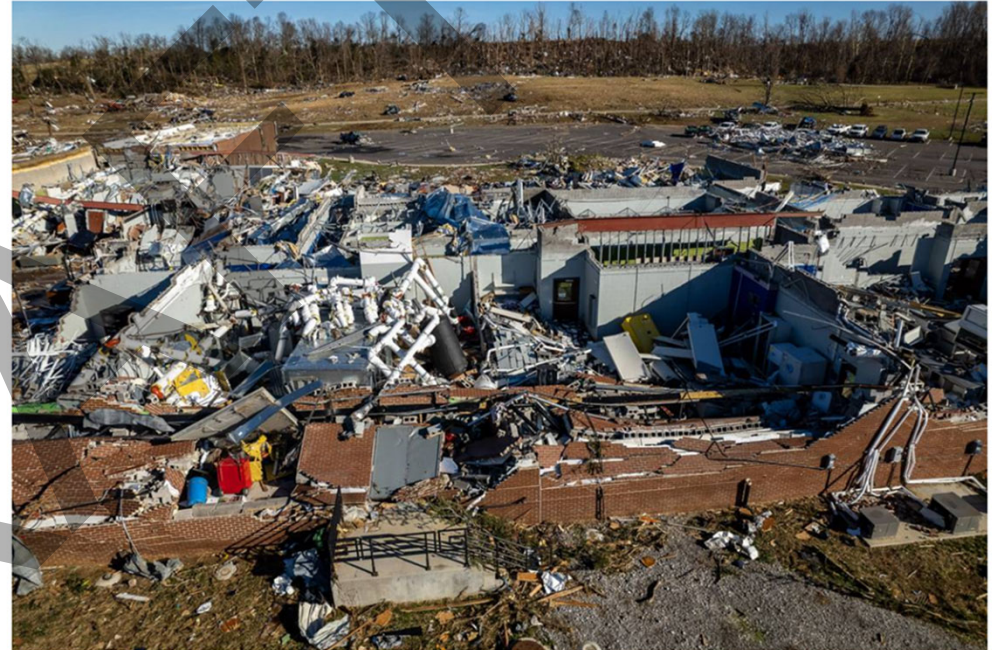
The Grain and Forage Center of Excellence at the University of Kentucky Research and Education Center in Princeton was damaged by a powerful tornado last weekend.. Matt Barton | UK College of Agriculture
