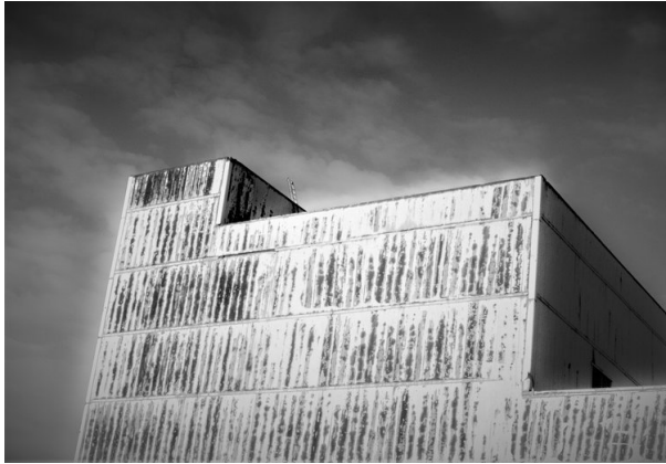
“Power House I”
