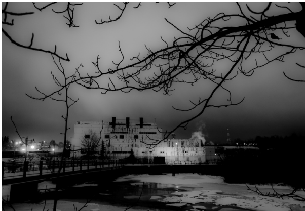
“Power House II”
