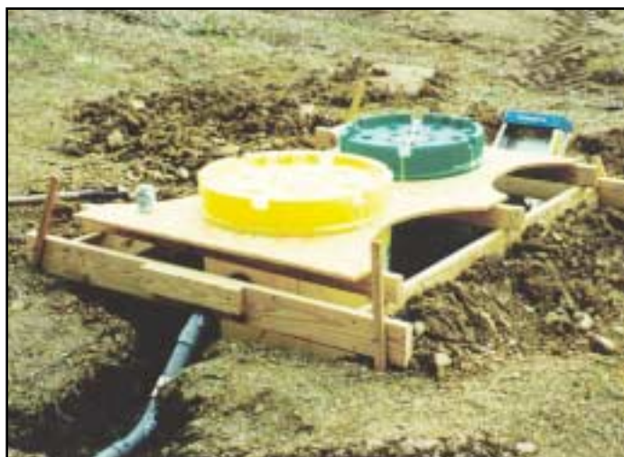
Figure 3b. Barrels in Positioning Jig. Notice conduit running to barrels.
