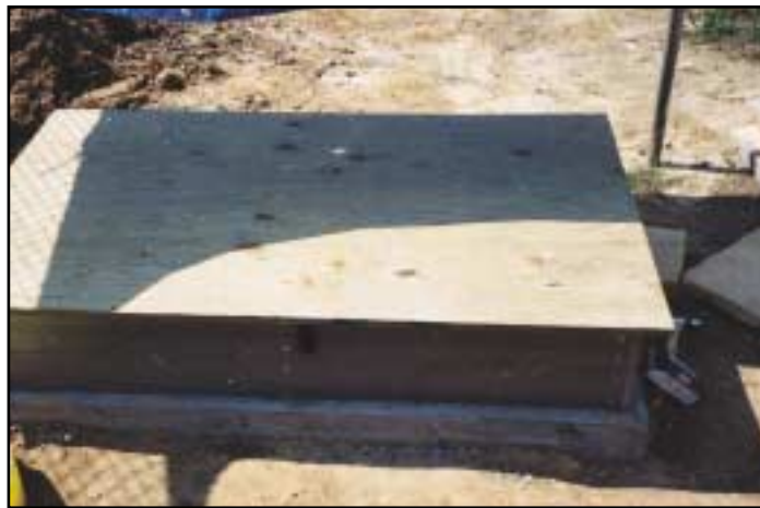
Figure 7. Vault door attached to frame.
