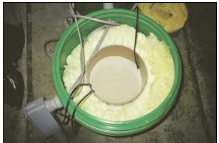
Figure 10c. Sand placement complete.
