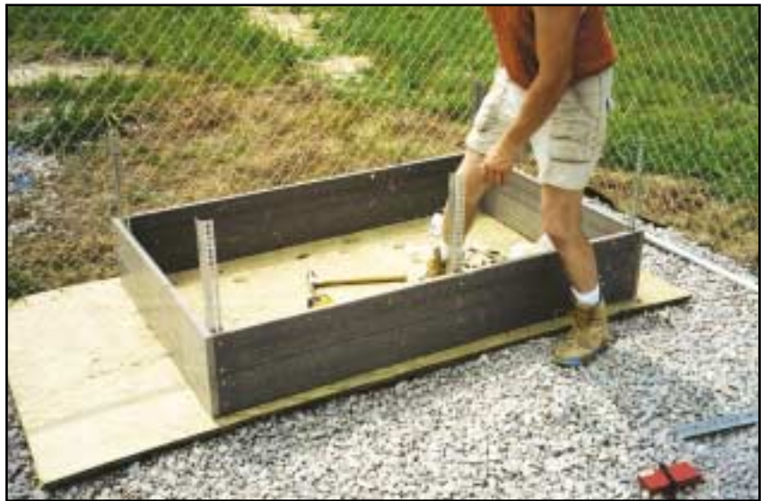
Figure 2. Assembling vault door frame.
