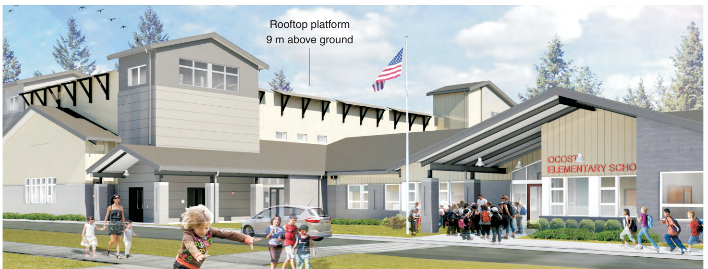
The four corner towers rose first (photo, July 2015). The completed tsunami refuge will span the flat roof of a gymnasium, with doors at ground level providing access through the corner towers (artist's conception).
