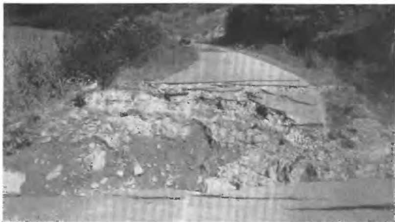
FIGURE 5.—Washed-out fill on State Route 5 at Jobs Run about 10 miles below Glenville. Courtesy of Corps of Engineers.
