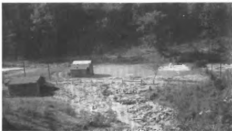
FIGURE 6.—Rock and mud deposit from a hillside wash. This wash drains about 2 acres in Right Fork Saltlick Creek basin. The man is standing at site of five-room house that was swept away by flood. Courtesy of Corps of Engineers.
