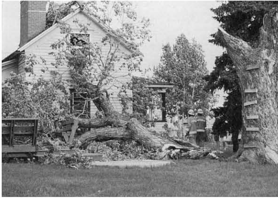
Plate 23.2 Photograph of one of several dozen houses in Fort Collins, Colorado, which sustained damage when large, fully-leaved trees were blown down by a moderately intense, out-of-season downslope windstorm on 3 July 1993. (Photograph by author)
