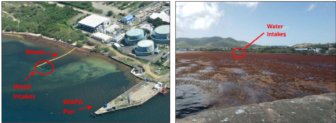
Figure 4-6. Aerial view of the WAPA plant and shoreline including the water intakes and initial booming strategy (yellow line), Sargassum on and near the beach (brown and orange colors), and the WAPA pier (left). A wider mass of floating Sargassum (orange colors) observed during the response, covering the water intakes and nearshore waters ~100 m or more from shore. Photo taken standing near the seaward end of the WAPA pier looking towards the water intakes and shoreline (right). Sources: Civil Air Patrol, FEMA.
