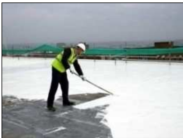
Figure 3: Creating a white roof is relatively simple
