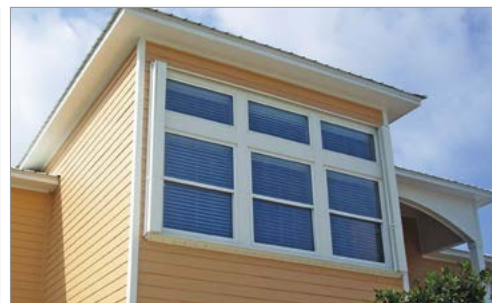
Figure 4-10. Accordion shutter (shown in the open position) installed over a large window of a coastal home. Shutter has been installed to allow deployment from inside the home. Image courtesy of Roll-a-way.
