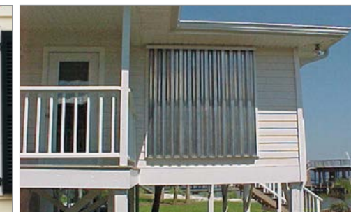
Figure 4-12. These 0.050 gauge aluminum storm panels offer cost effective storm protection. In this example, panels slip into a track above the window and secure onto a bottom track using wing nuts.
