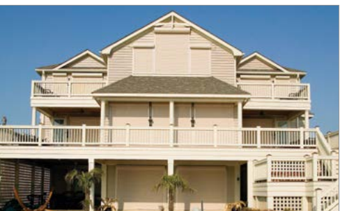
Figure 4-9. Coastal home protected with roll-down shutters on all windows and doors. The shutter is held in place by vertical guide tracks and can be deployed manually or with an integrated electric motor. Image courtesy of QMI, Inc.
