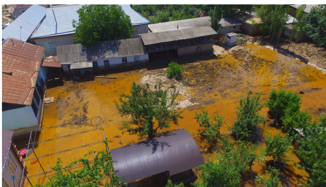
Flooded site. Drone image, MES, T.K.Izabekov
