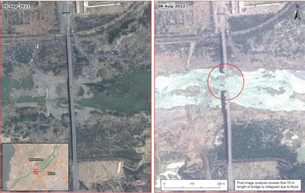
Hub River Bridge on N-25, Lasbela
