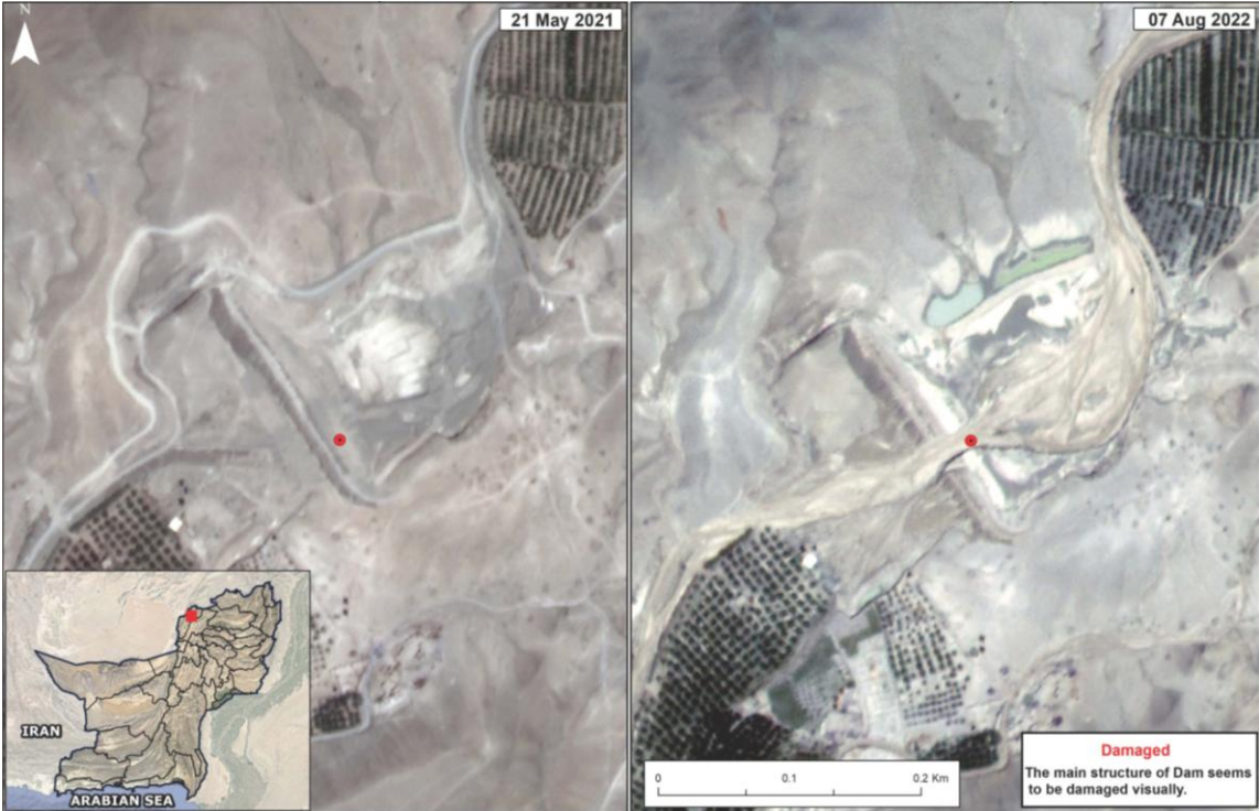
Dam Breach – Qilla Abdullah, Balochistan
