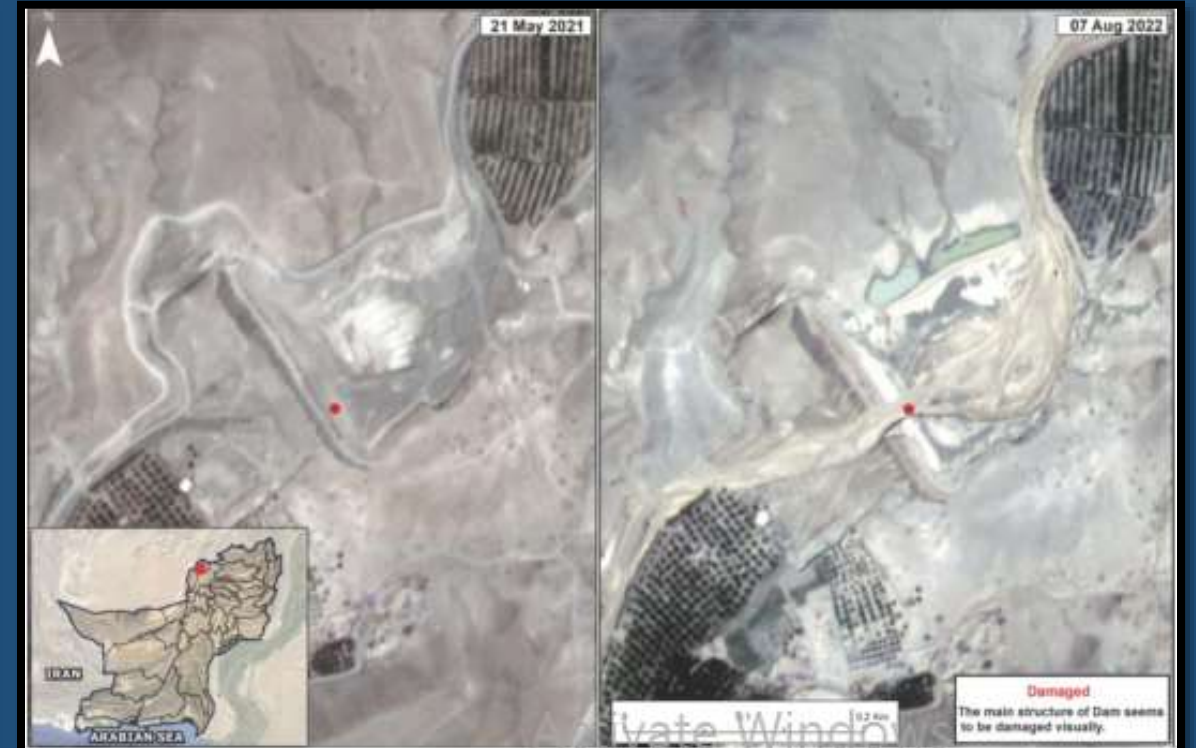
Dam Breach - Qilla Abdullah , Balochistan
