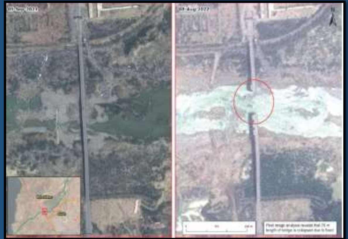
Hub River Bridge on N-25 Lasbella
