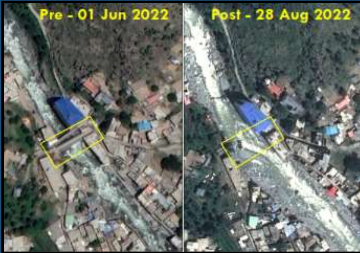
Collapsed Bridge on N-35
