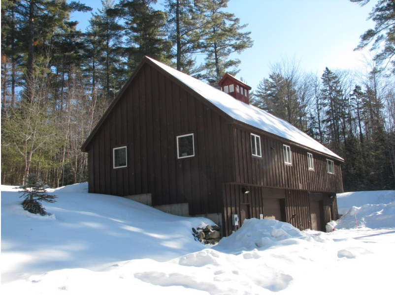
Ranger's residence/maintenance building on Little Pond Road
