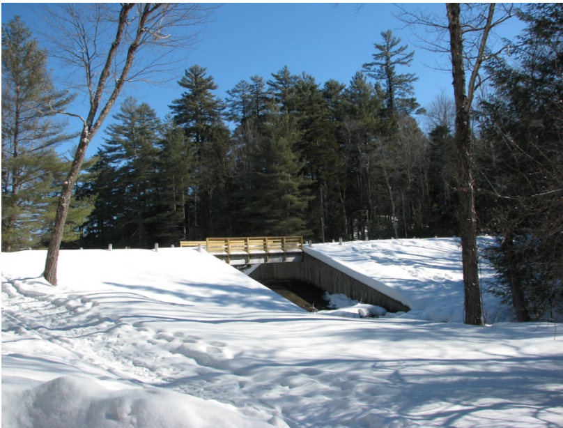
Lowell Lake dam and bridge
