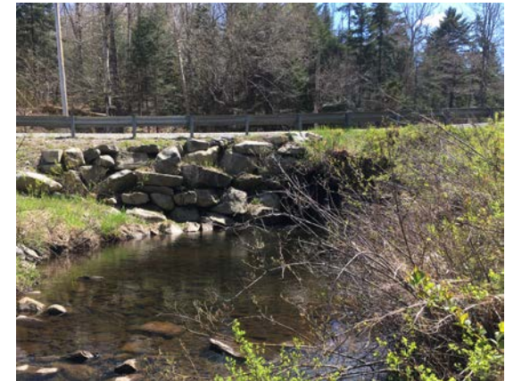
Downstream end of culvert
