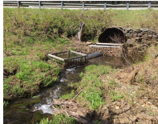
Upstream end of culvert
