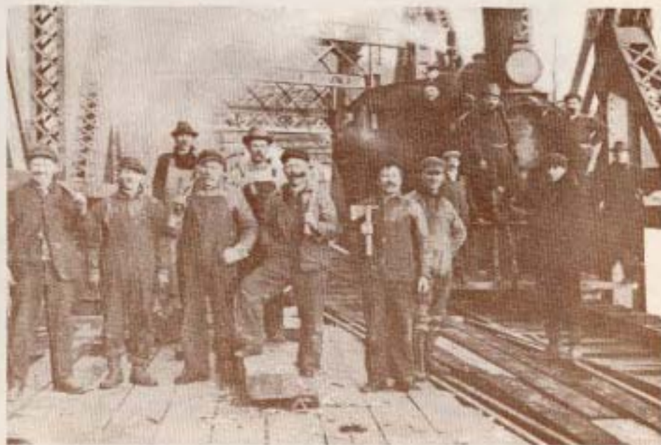
Construction Crew 1910. BP
