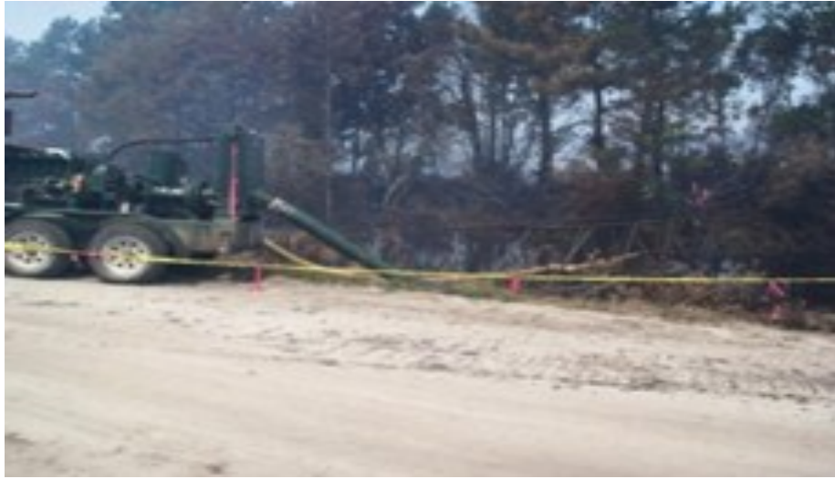
Water pumping operations at the Dad Fire
