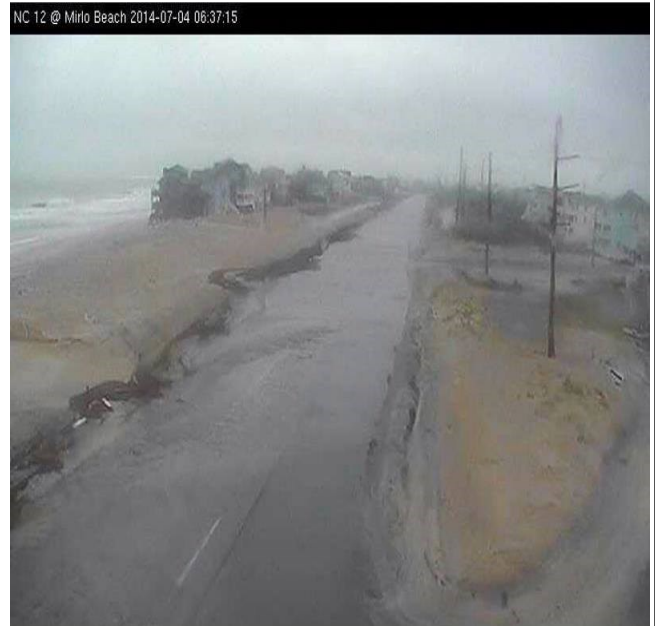
Overwash on Highway 12 at Mirlo Beach Courtesy NC Department of Transportation
