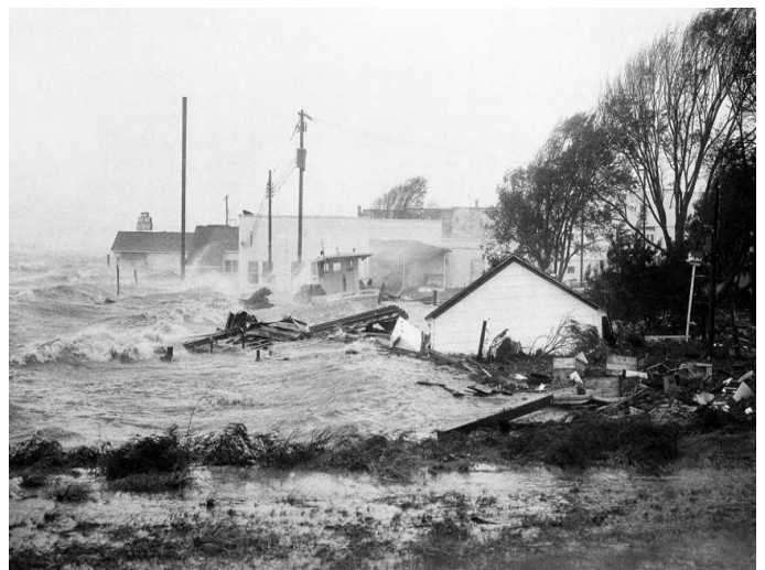
Severe Surge Flooding in Morehead City
