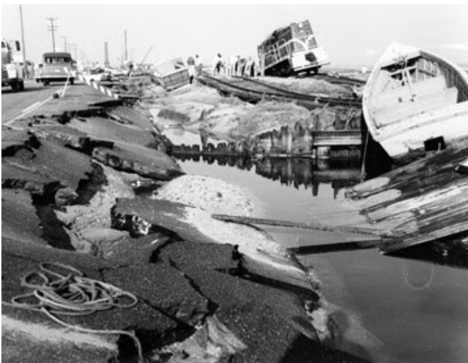
Damage to the Beaufort-Morehead City Causeway
