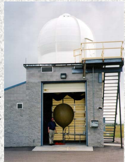
Upper air building. Tracking dish is inside the dome on top. Balloon is inflated inside.
