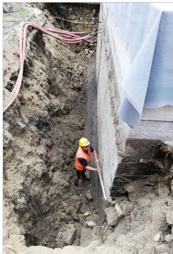
Waterproofing the foundation of the Montfaucon Monument, France
