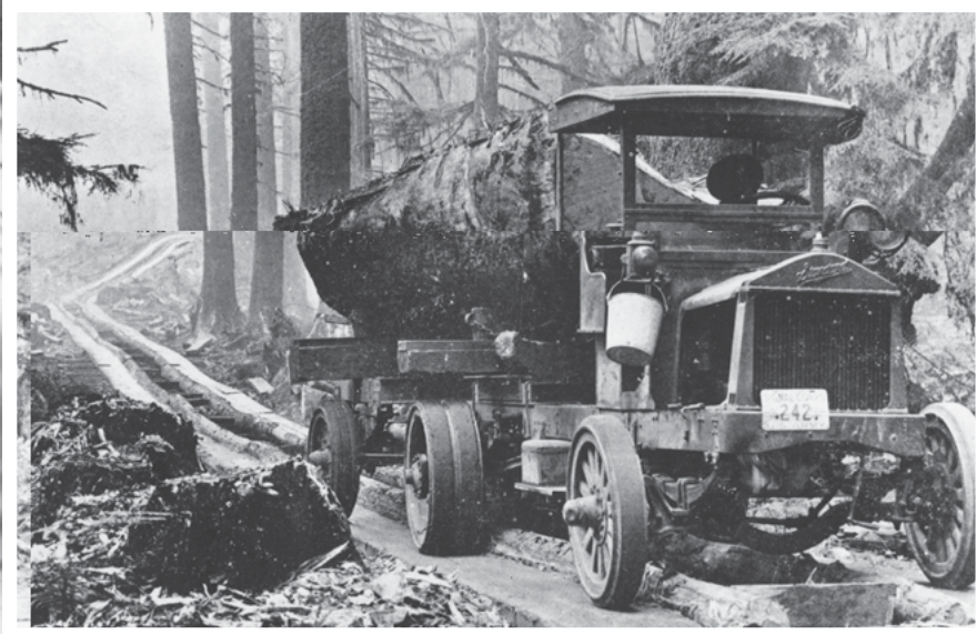
An Army truck at work in the Spruce Production Division's logging in the Northwest.
