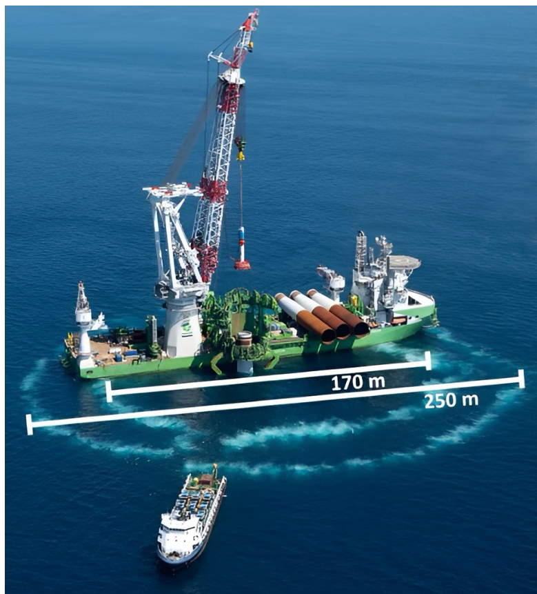
Bubble curtains are used during monopile foundation installation to, minimizing acoustic impacts to fish and protected species. Double bubble curtains are especially effective and can lower sound energy levels by up to 90%. Credit: DEME Group
