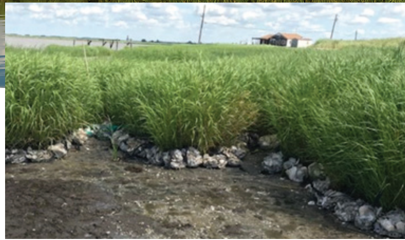
Left: Clump of oysters collected from a restoration site planted with recycled oyster shells. Photo credit: NJ Fish and Wildlife Shell Recycling Program. Right: Bags of recycled oyster shells are set around Spartina marsh to protect against erosion. Photo (c) Long Beach Township Shell Recycling Program.
