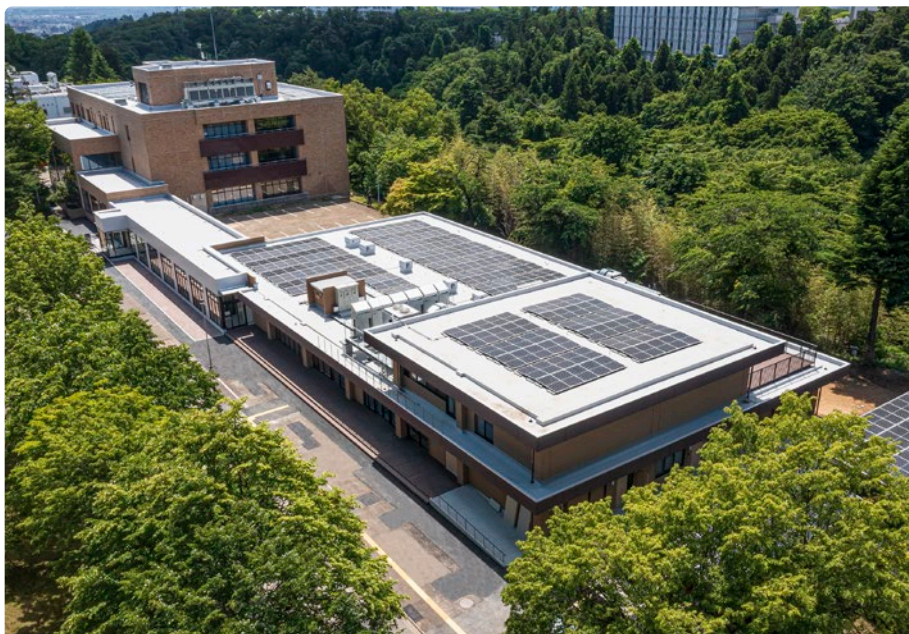
Kita-Aobayama Center Square (completed in May 2023)
