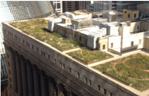
Figure III-5. Roof of Chicago City Hall
