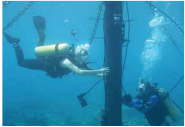
Figure 37: Stringing underwater cables on a Coral Reef Early Warning System station. Credit: NOAA
