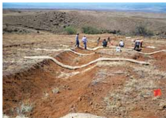
Figure 55: Project staff installing erosion control fabric in the watershed. Photo credit: Kohala Watershed Partnership
