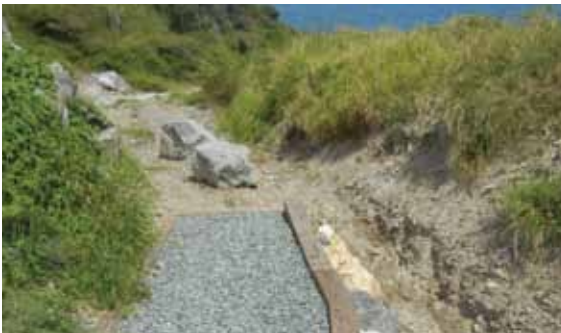
Figure 64: Trail stabilization technique at East End Bay. Photo credit: NOAA
