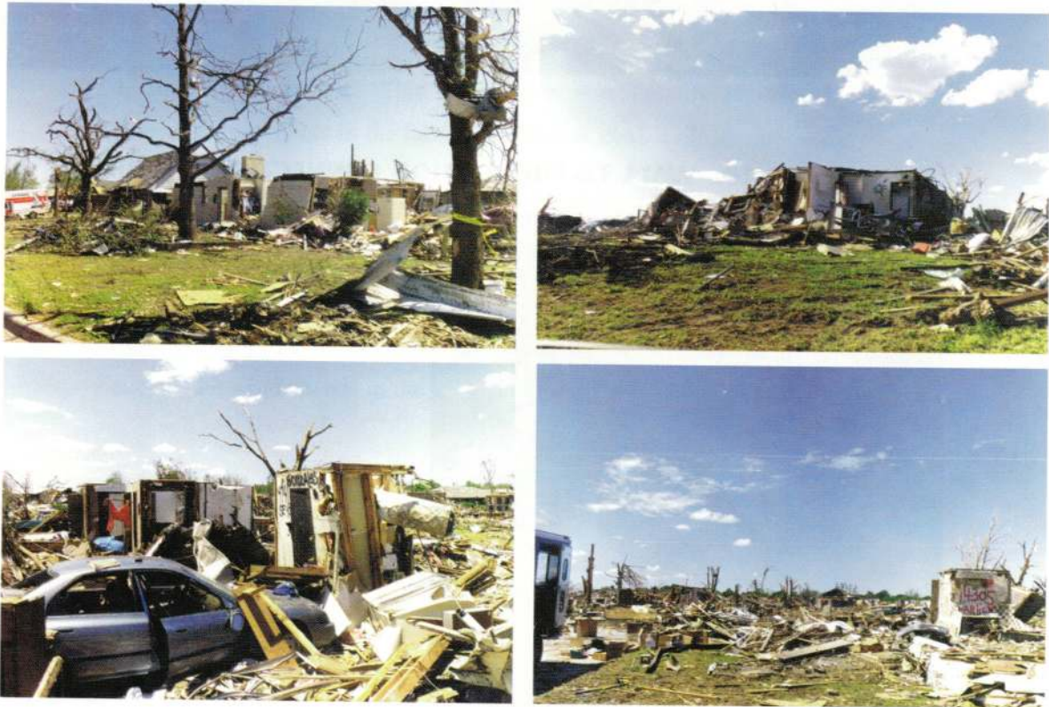
FIGURE 8. SEVERE DAMAGE (F3 DAMAGE LEVEL)
