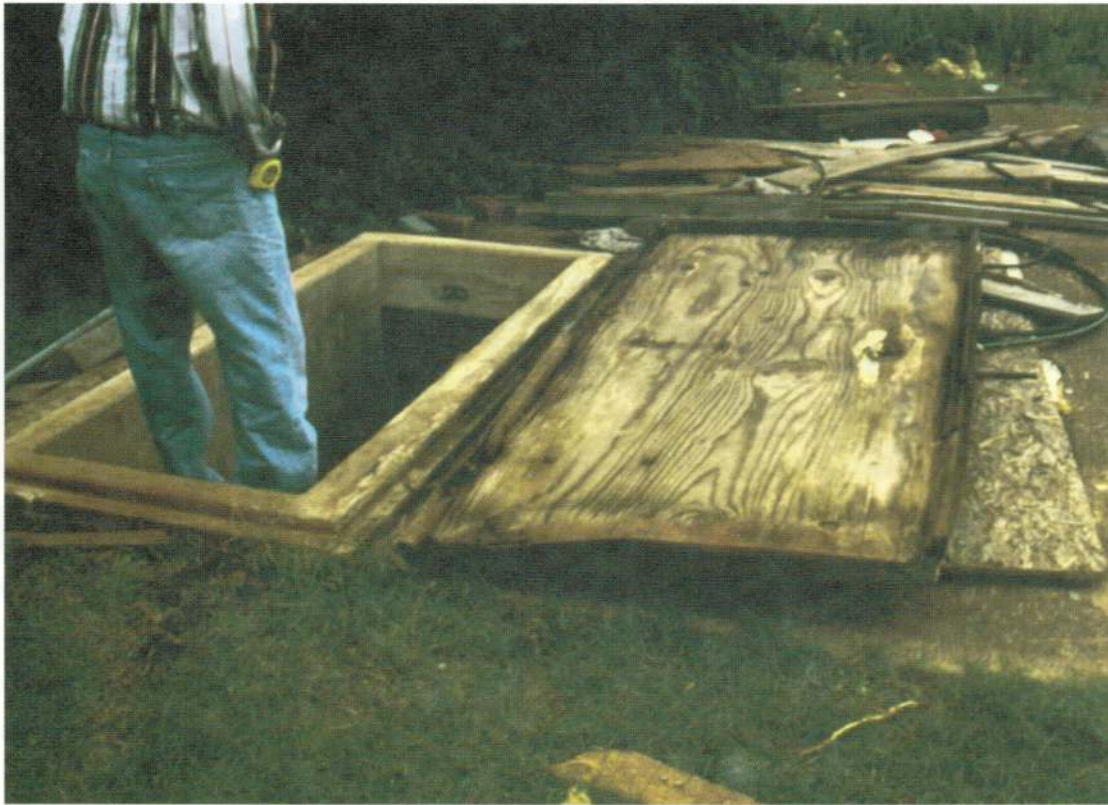
FIGURE 18. BRIDGE CREEK CELLAR DOOR
