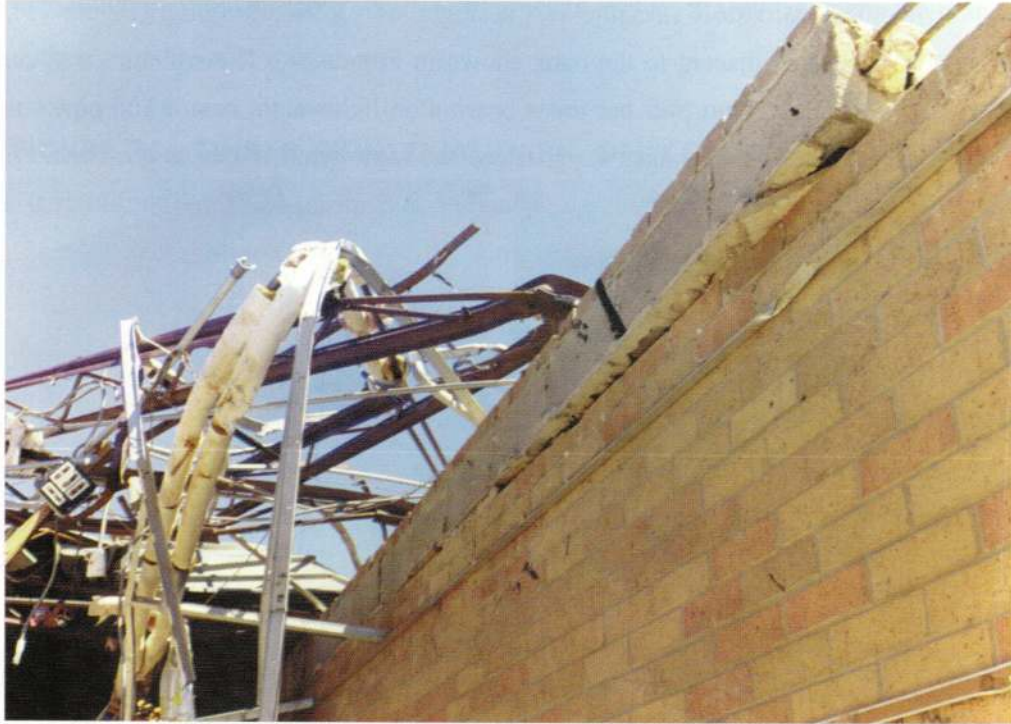
FIGURE 23. KELLY ELEMENTARY, MASONRY BEARING WALL
