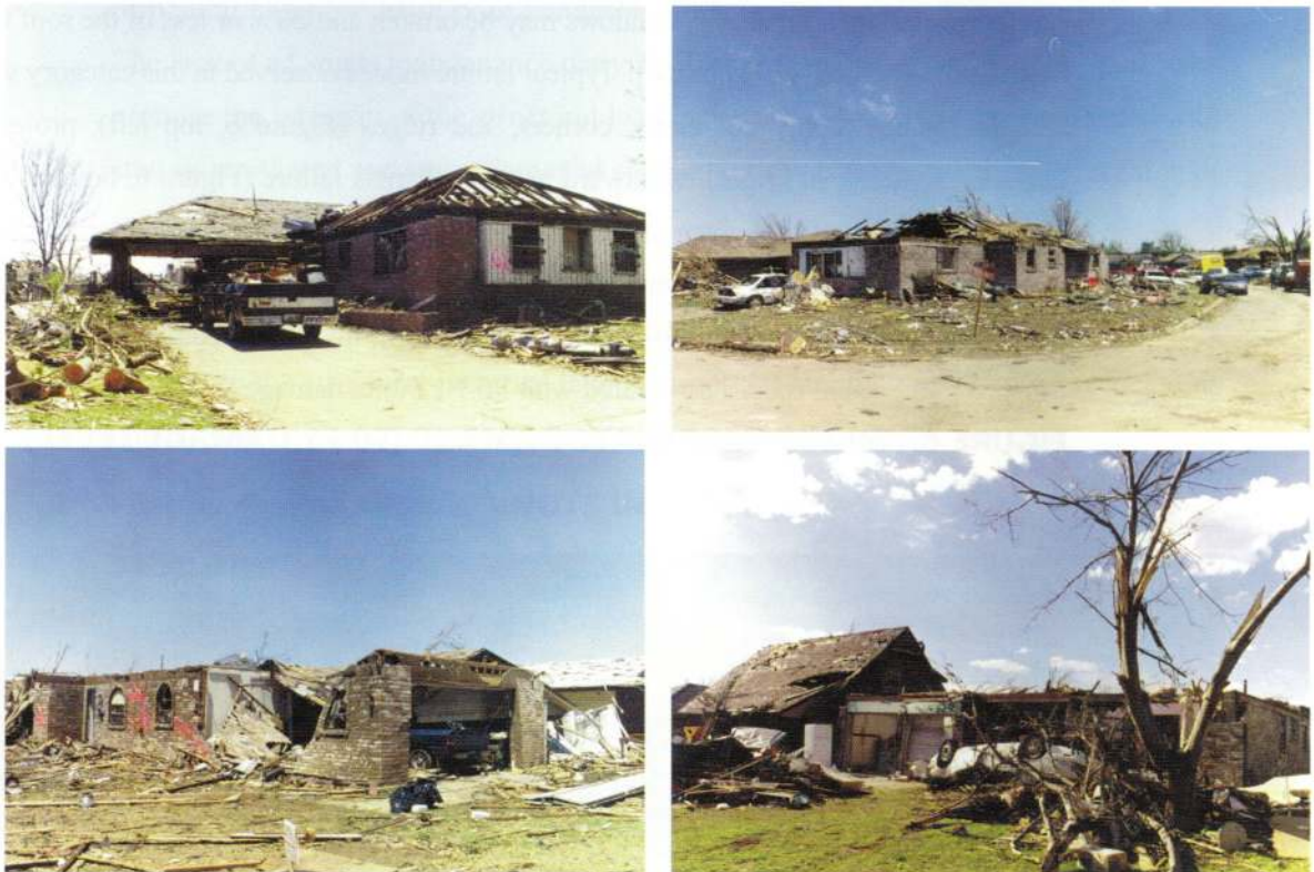
FIGURE 7. EXTENSIVE DAMAGE (F2 DAMAGE LEVEL)
