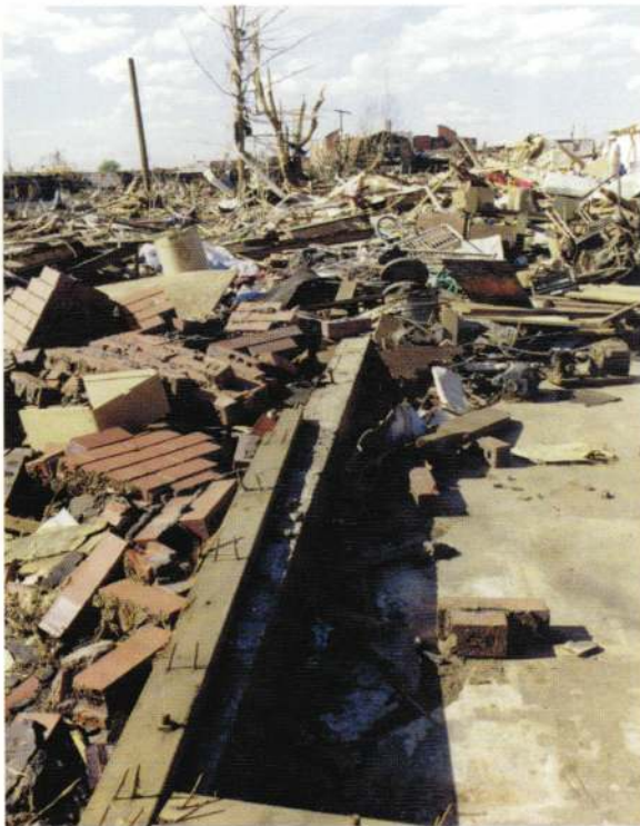
FIGURE 10. WALL TO FOUNDATION CONNECTION FAILURE
