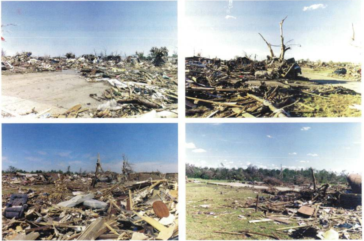
FIGURE 9. DESTROYED (F4-F5 DAMAGE LEVEL)
