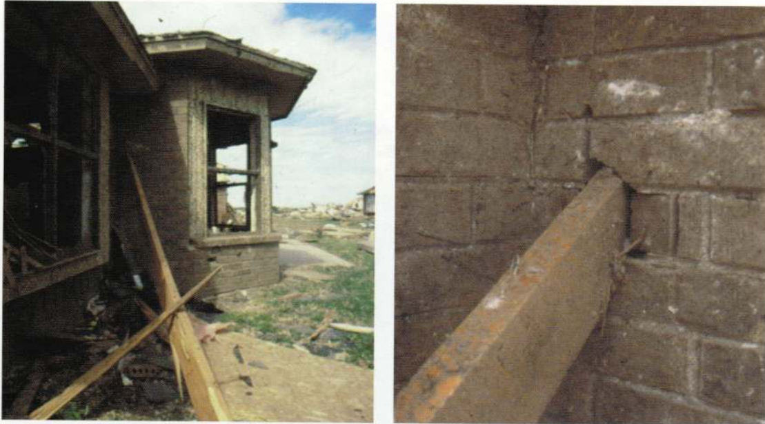
Figure 32. Large 2x6 Wood Projectile
