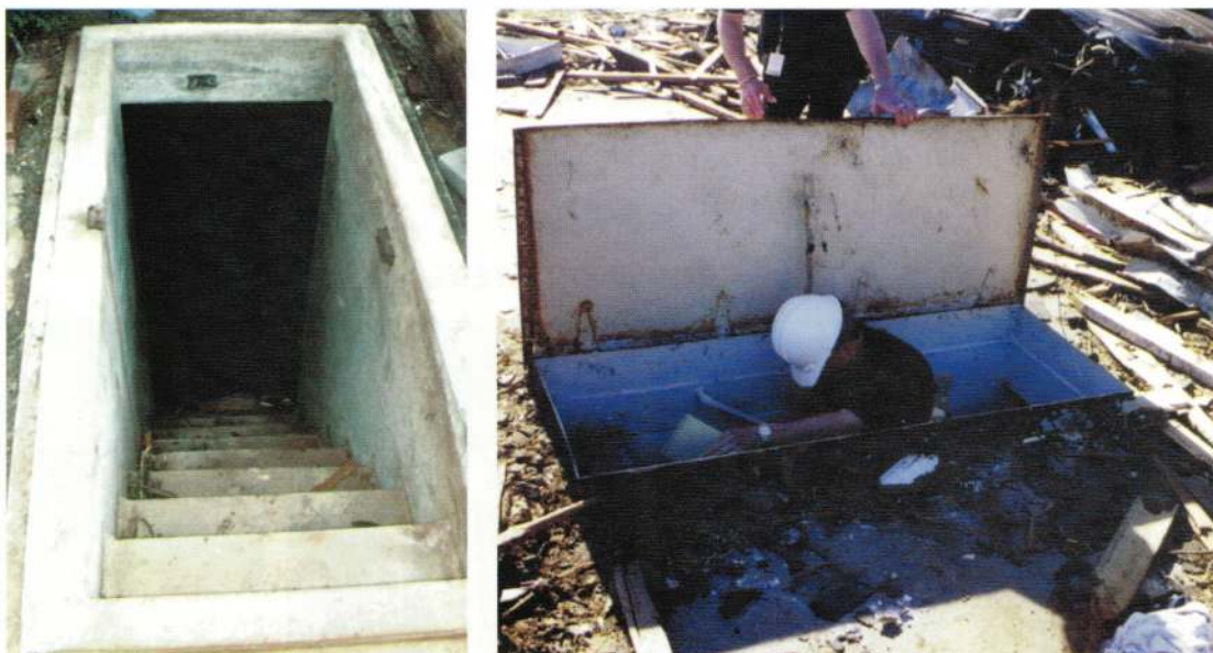
Cast-in-place concrete (left); prefabricated steel (right).
