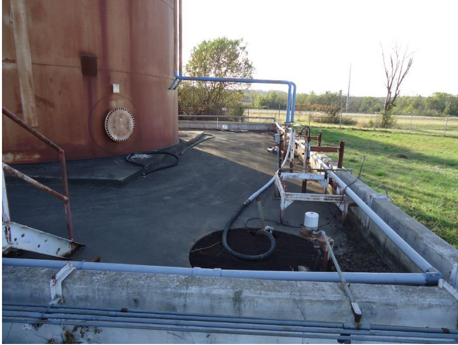
Tank V-68 secondary containment and sump
