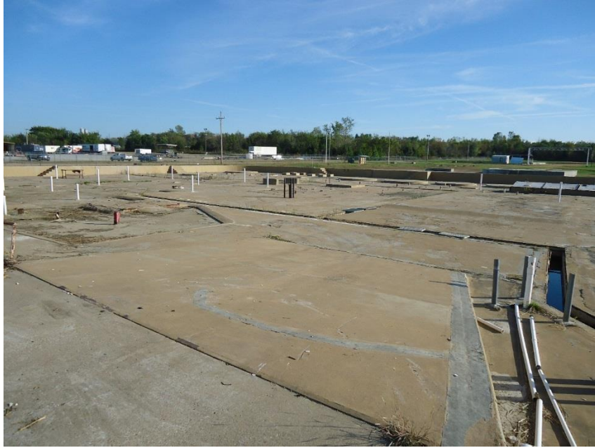
Former solvent recycling plant view towards the southeast
