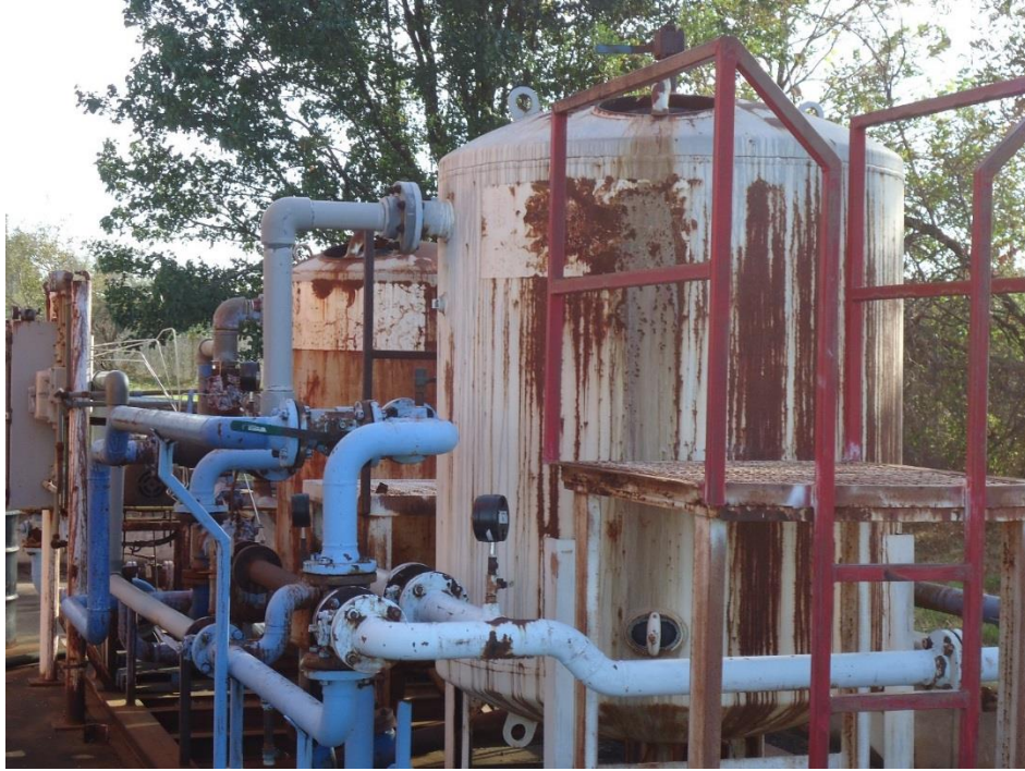
Water treatment carbon bed
