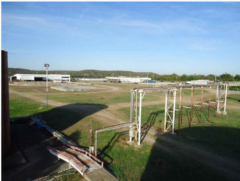
View to the Northeast from top of Tank V-69
