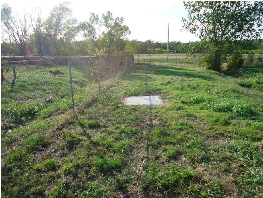
Recovery Sump #2 outside facility north fence (outer collection trench)
