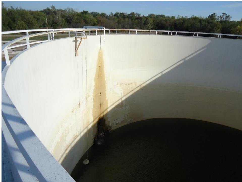
Inside view of groundwater collection pipe into double walled open top tank
