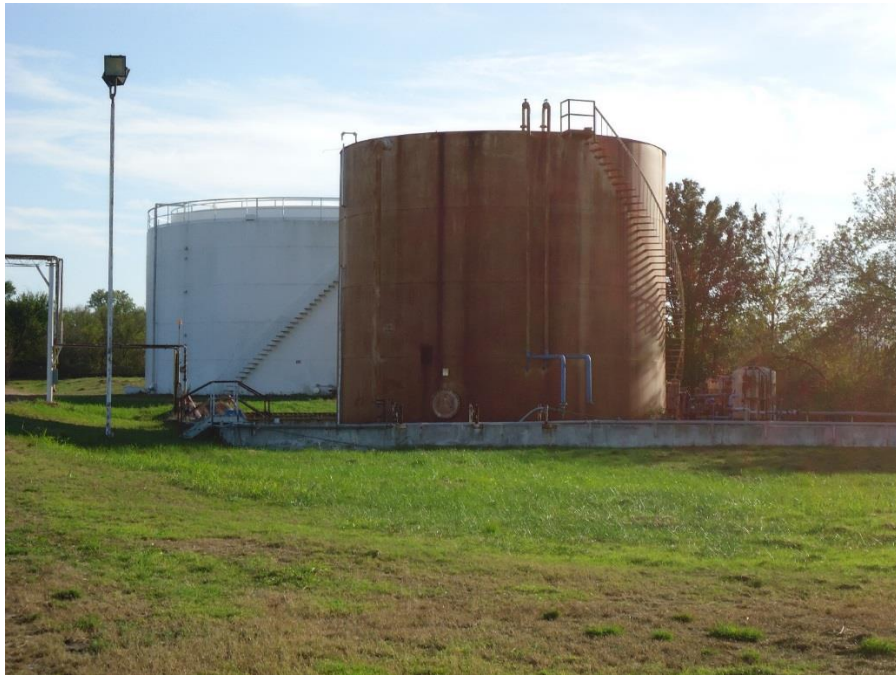
Tank V-68 (foreground) and Tank V-69 (background)
