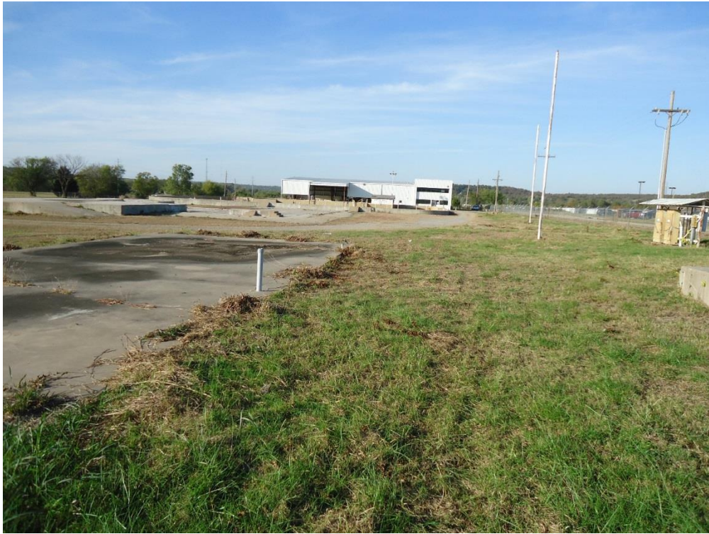
View of facility from the South facing North
