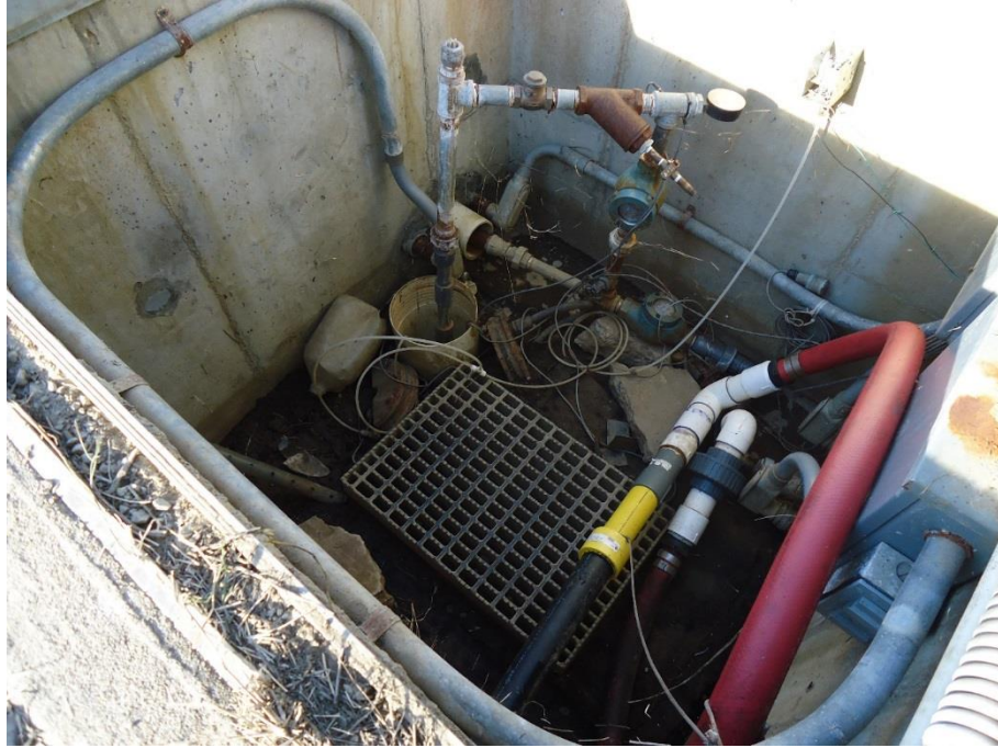
Inside of Recovery Sump #4
