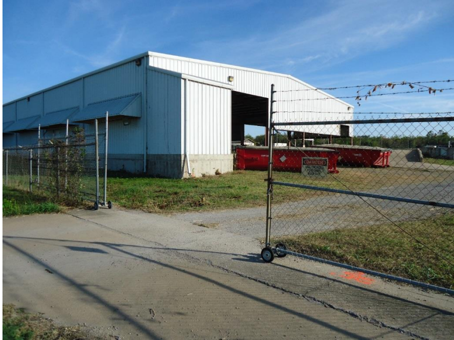
North entry gate facing southeast and North drum storage pad under roof
