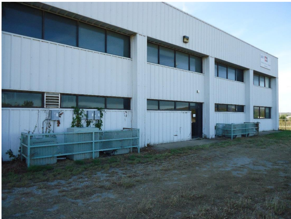
Main facility building entrance
