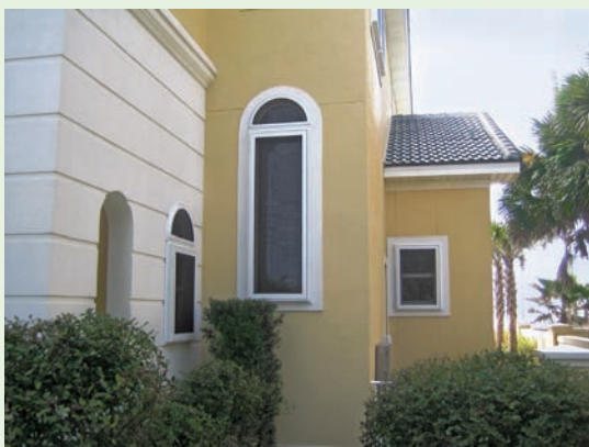
Figure 4-15. In-place stainless steel impact screen protects several windows of a coastal residence. This system requires no deployment and provides shade. Image courtesy of Roll-a-way
