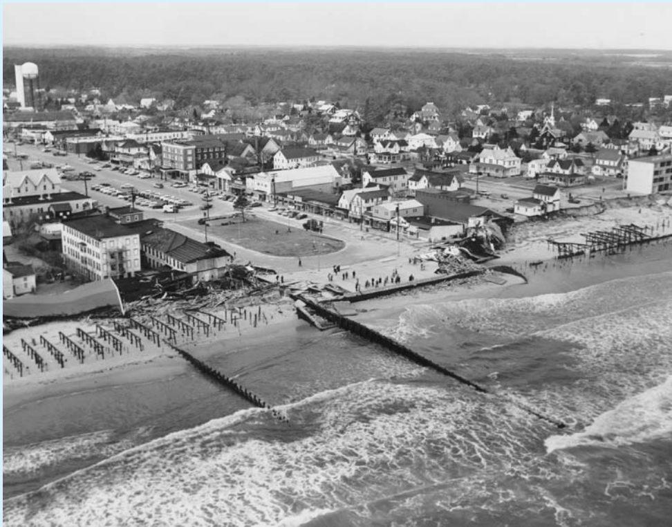
Figure 2-5. The March 1962 northeaster caused significant damage to property in Delaware, especially along the coastlines of the Inland Bays, Delaware Bay, and Atlantic Ocean. Image courtesy of Delaware Public Archives
