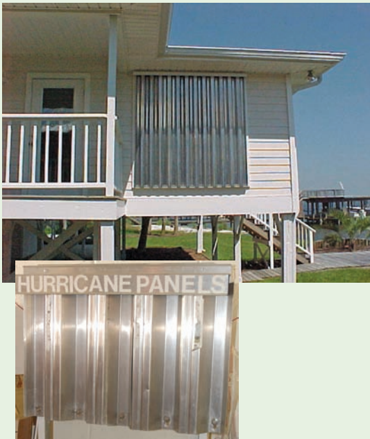
Figure 4-14. These 0.050 gauge aluminum storm panels offer cost effective storm protection. In this example, panels slip into a track above the window and secure onto a bottom track using wingnuts. Image courtesy of Roll-a-way
