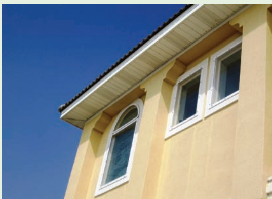
Figure 4-16. Flat impact polycarbonate panels are installed directly over windows of a coastal home. This window covering provides excellent storm protection with minimal aesthetic impact. Image courtesy of Roll-a-way
