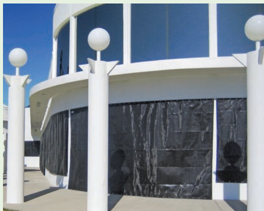
Figure 4-17. Polyethylene basketweave fabric windscreen deploys directly over ground floor windows of a coastal home. Image courtesy of Roll-a-way
