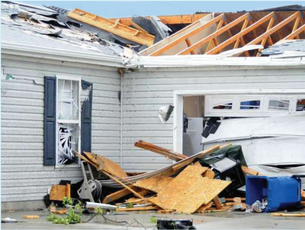
Figure 2-11. In September 2012, an EF-0 tornado with estimated maximum wind speeds of 85 mph caused structural damage in Kent County, Del. Image courtesy of Kent County Office of Emergency Management
