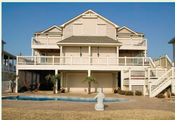
Figure 4-11. Coastal home protected with roll-down shutters on all windows and doors. The shutter is held in place by vertical guide tracks and can be deployed manually or with an integrated electric motor. Image courtesy of QMI, Inc.
