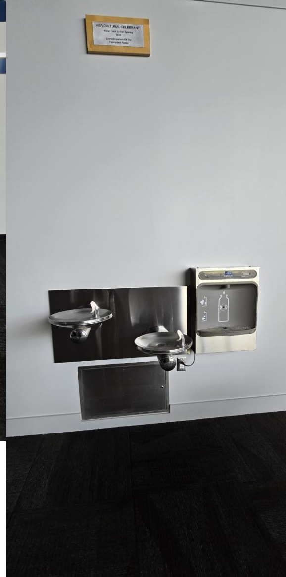
High/Low Water Fountains. Lowered Bottle Fill Station.
