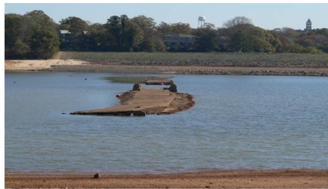
MEMORIAL BRIDGE (Photo courtesy of Mr. Doug Young)
