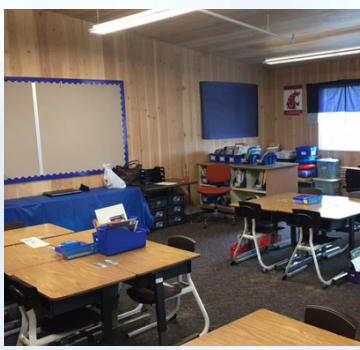
One of four cross-laminated timber classrooms built at Adams Elementary in the Wapato School District.
