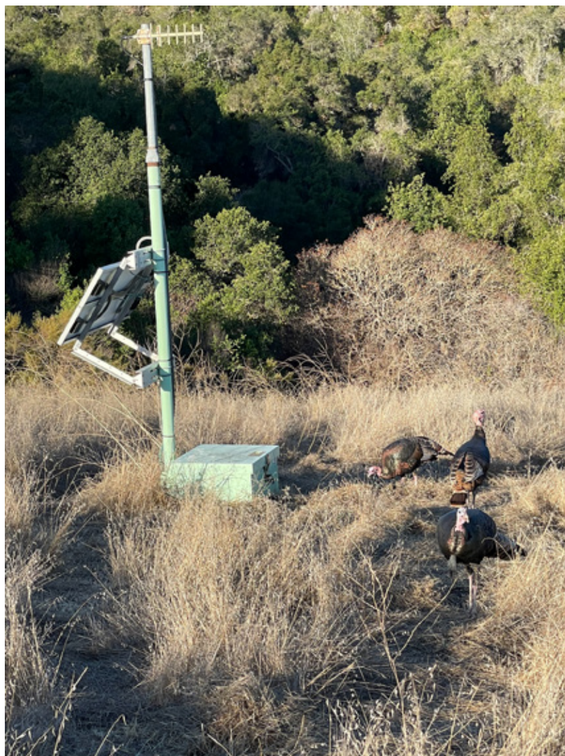
Earthquake early warning system monitoring station.
