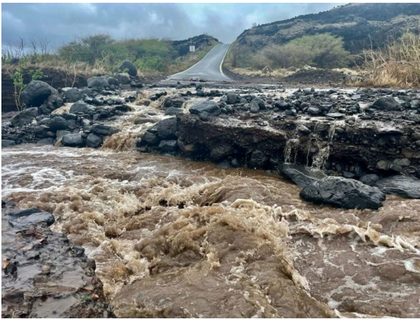
Flooded roadway at Nu'u, Kaupō Gap, Maui. Source: Maui Police Department.
