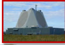
Force protection and vulnerability assessments of national and allied infrastructure
