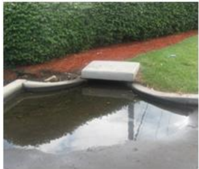
Figure 46. Water with sheen and brown foam; Water pooling around drain
