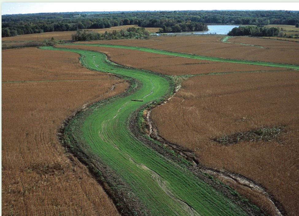
A grassed waterway system is one tool to prevent soil erosion by reducing water flow velocities.
