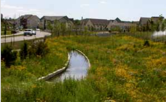
FIGURE 5-57 View of a sediment trap and porous landscape detention area in the central parkway spine of Heritage Park. The sediment trap in the center left of the photo was designed for ease of maintenance access by city crews with standard city maintenance equipment. Courtesy of SRF Consulting Group, Inc.
