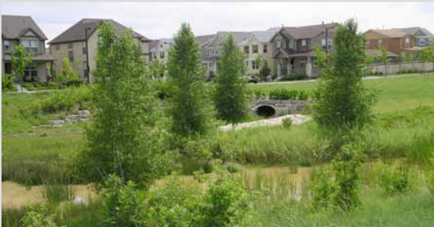
FIGURE 5-56 A consolidated treatment area adjacent to one of several neighborhoods that have been constructed as part of the project's build-out.
