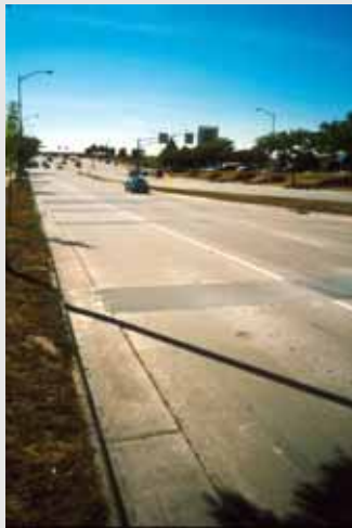
Wide arterial street with little roadside vegetation
