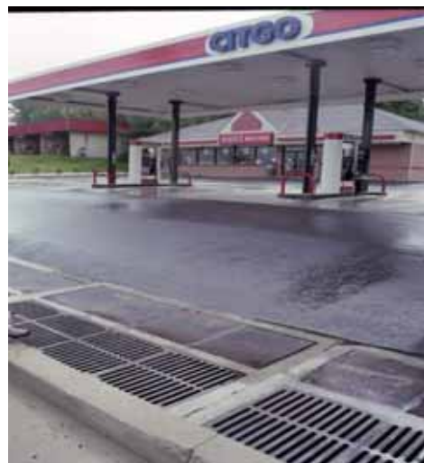
FIGURE 5-46 Delaware sand filter. SOURCE: Tom Schueler.
