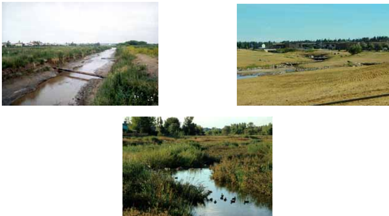
FIGURE 5-48 Three photographs illustrate stream rehabilitation in Denver. The top left picture is a creek that has eroded in its bed due to urbanization. The top right picture shows a portion of the stabilized creek immediately after construction. Check structures, which keep the creek from cutting its bed, are visible in the middle distance. The bottom image shows the creek just upstream of one of the check structures two years after stabilization. The thickets of willows established themselves naturally. The only revegetation performed was to seed the area for erosion control.
