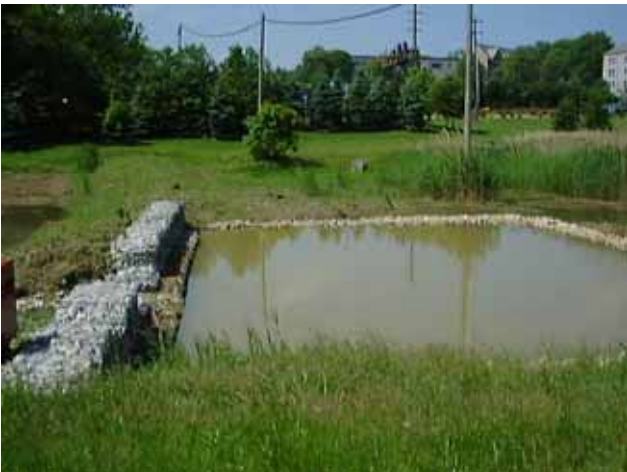
FIGURE 5-44 Villanova University sediment forebay. SOURCE: Reprinted, with permission, from VUSP. Copyright by VUSP002E
