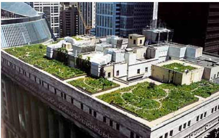
FIGURE 5-18 City Hall in the center of Chicago's downtown was retrofitted with a green roof to reduce the heat island effect, remove airborne pollutants, and attenuate stormwater flows as a demonstration of innovative stormwater management in an ultra-urban setting. SOURCE: Conservation Design Forum.
