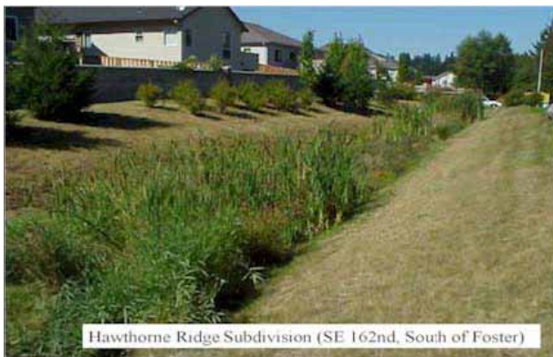
FIGURE 5-16 Vegetated swale. SOURCE: PaDEP (2006).
