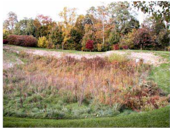
FIGURE 5-43 Dry extended detention pond. SOURCE: PaDEP (2006).
