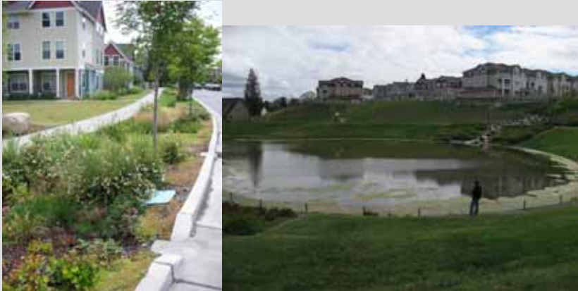
FIGURE 5-58 Natural drainage system methods have been applied to a 34-block, 1,600-unit mixed-income housing redevelopment project called High Point. Vegetated swales, porous concrete sidewalks, and frontyard rain gardens convey and treat stormwater on-site. On the right is the detention pond for the development.
