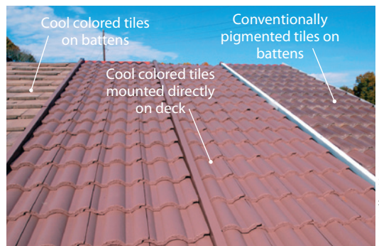
Figure 8: Conventional and Cool Colored Tiles
