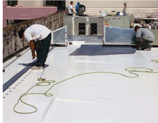
Figure 14: Installation of a Cool Single-Ply Membrane
