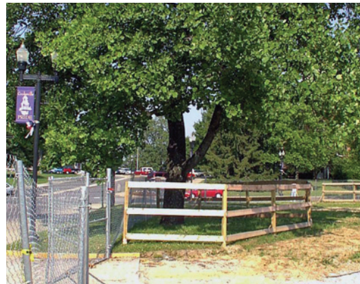
Figure 4: Fences Protect a Tree During Construction
