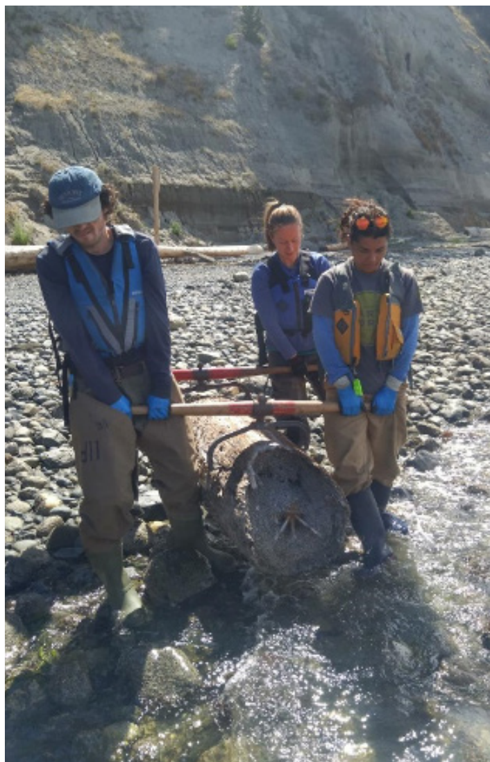
A creosote piling being removed from Lopez Island, WA.
