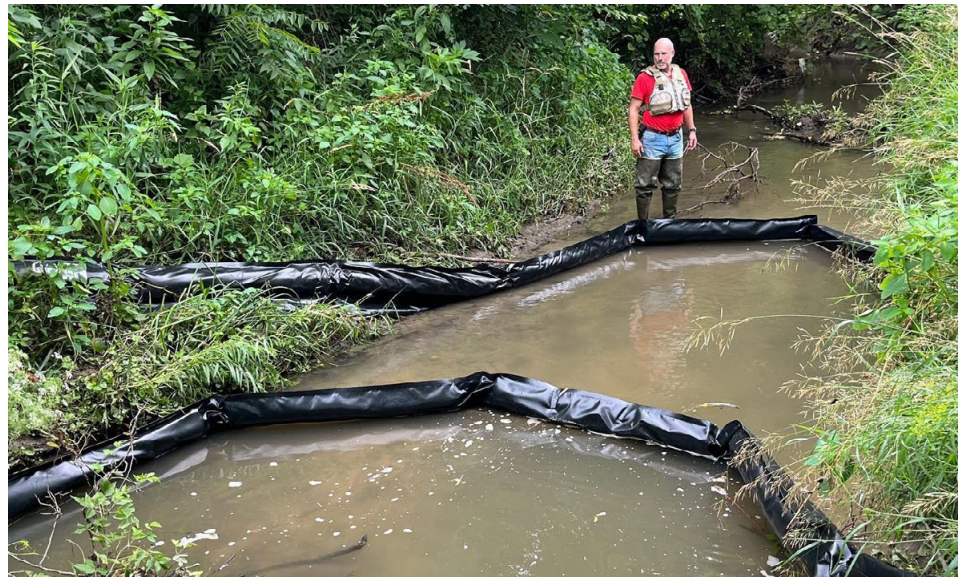
Osprey Initiative installing a litter boom in a local Davenport creek.
