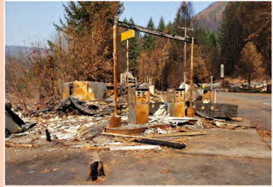
The Rivers Run facility after it was destroyed by the Lionshead fire
