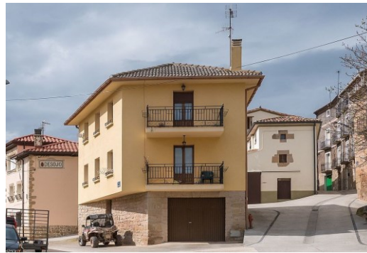
brick masonry mass wall structure
