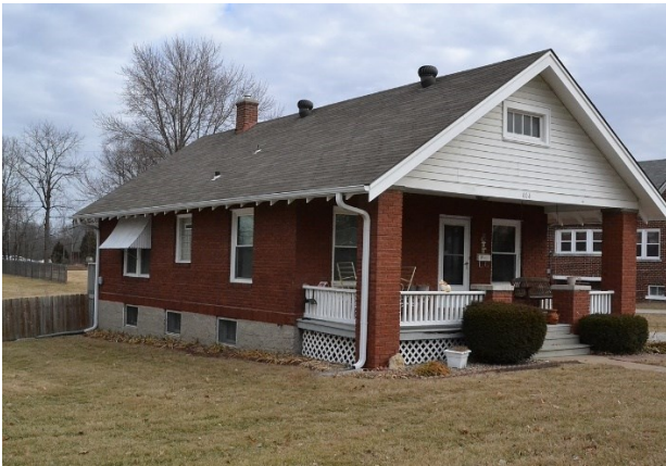
weak wooden frame structure with brick veneer
