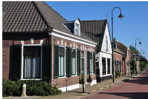
brick masonry mass wall structure
