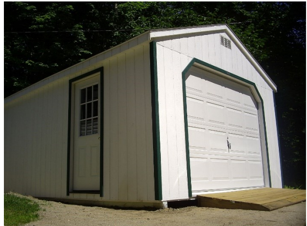
metal frame structure with wooden panels
