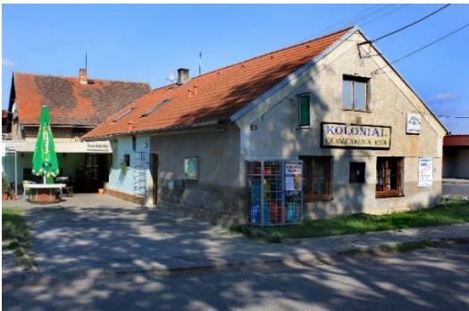
concrete block mass wall structure
