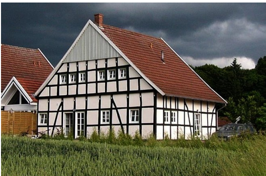
strong wooden frame structure
