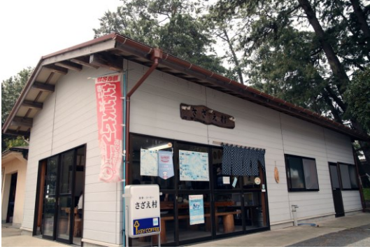
strong wooden frame structure
