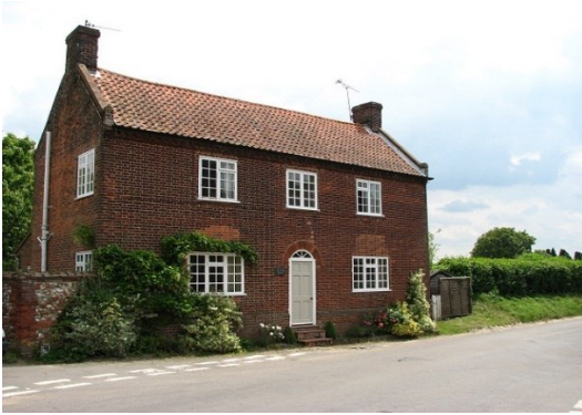
brick masonry mass wall structure
