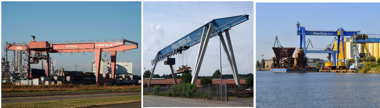
Figure 3-1. Container / gantry cranes
