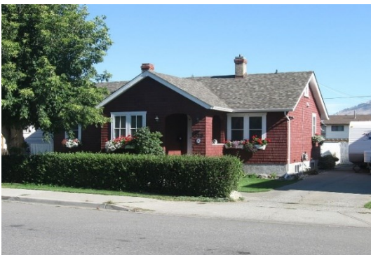
strong wooden frame structure with brick veneer
