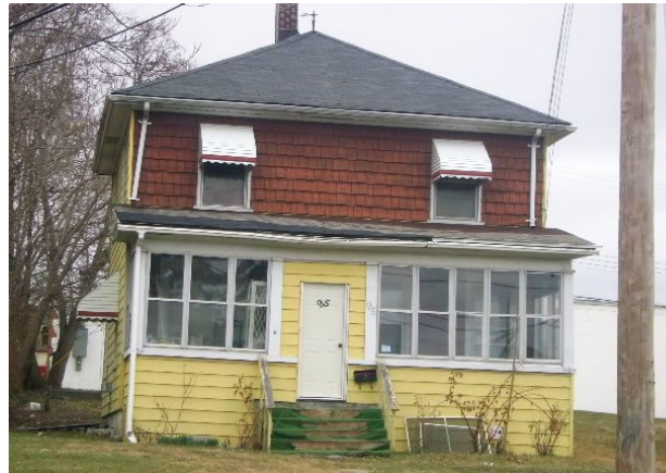
weak wooden frame structure
